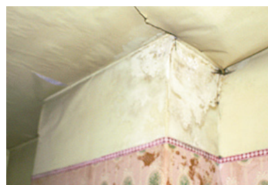
▲ Internal penetrating damp
